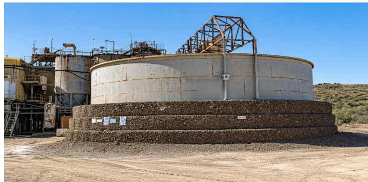
Bamboo Creek Processing Plant Thickener
