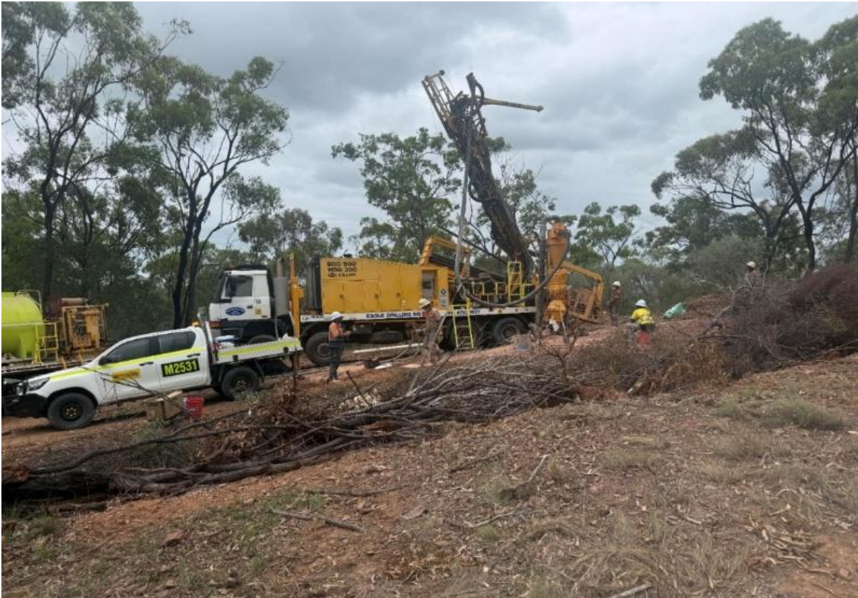
Figure 1: Drilling at Podoskys
