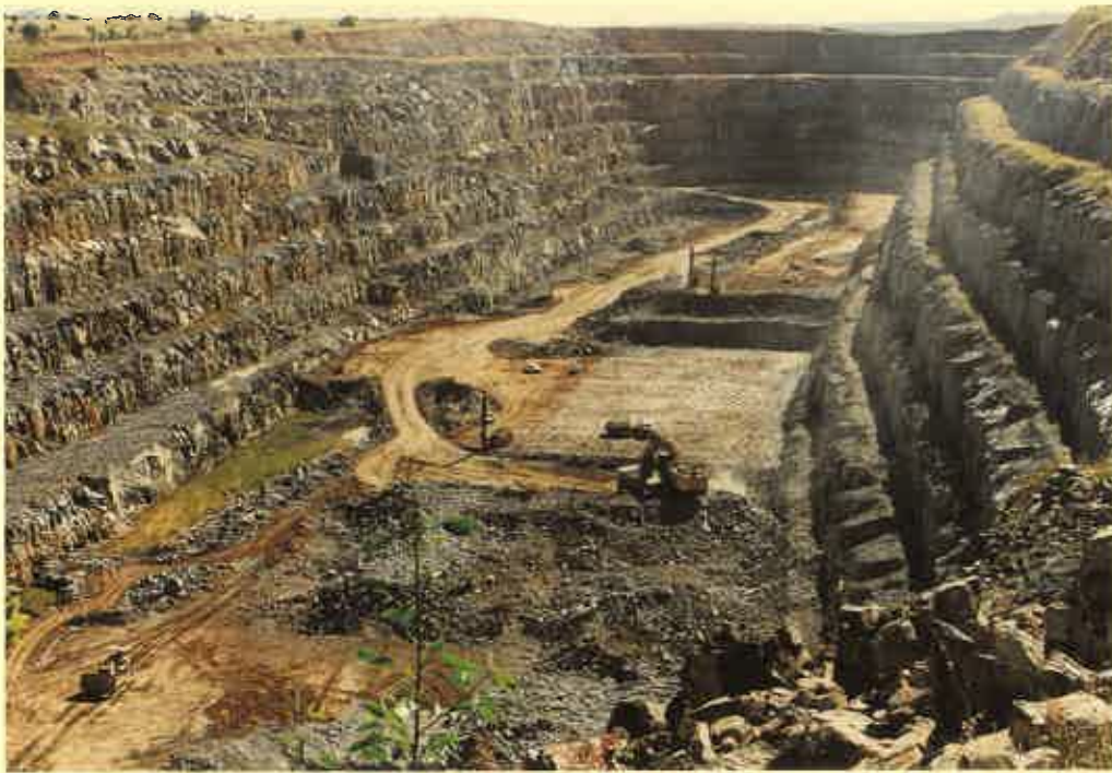
Nolans Pit looking west (preparation for blasting)
