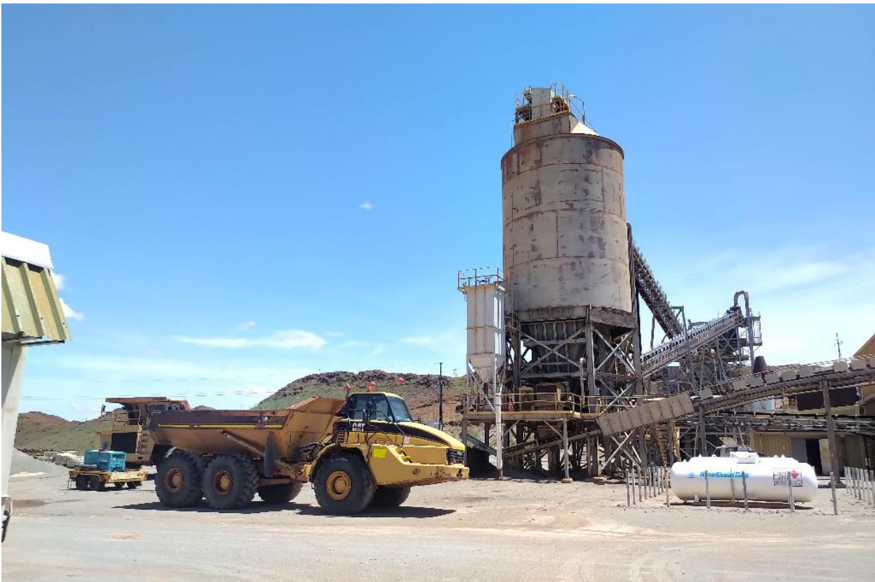
Figure 2: Bamboo Creek Pilot Plant
