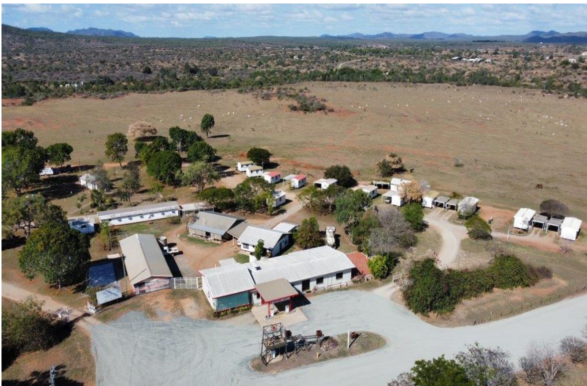
Figure 20: Aerial view of Haoma's Top Camp, Ravenswood, Queensland.
