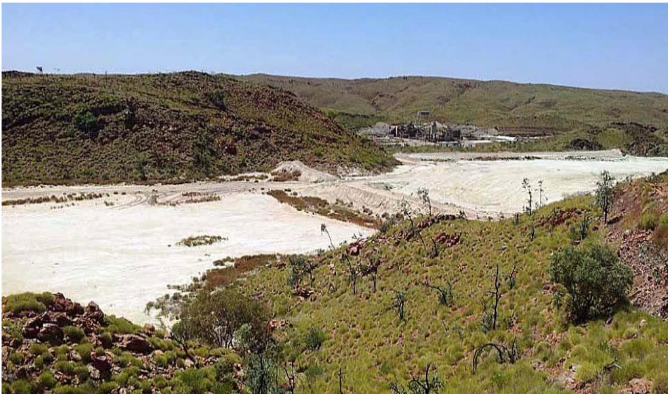
Figure 3: Bamboo Creek Tailings Storage with Bamboo Creek Processing Plant in background
