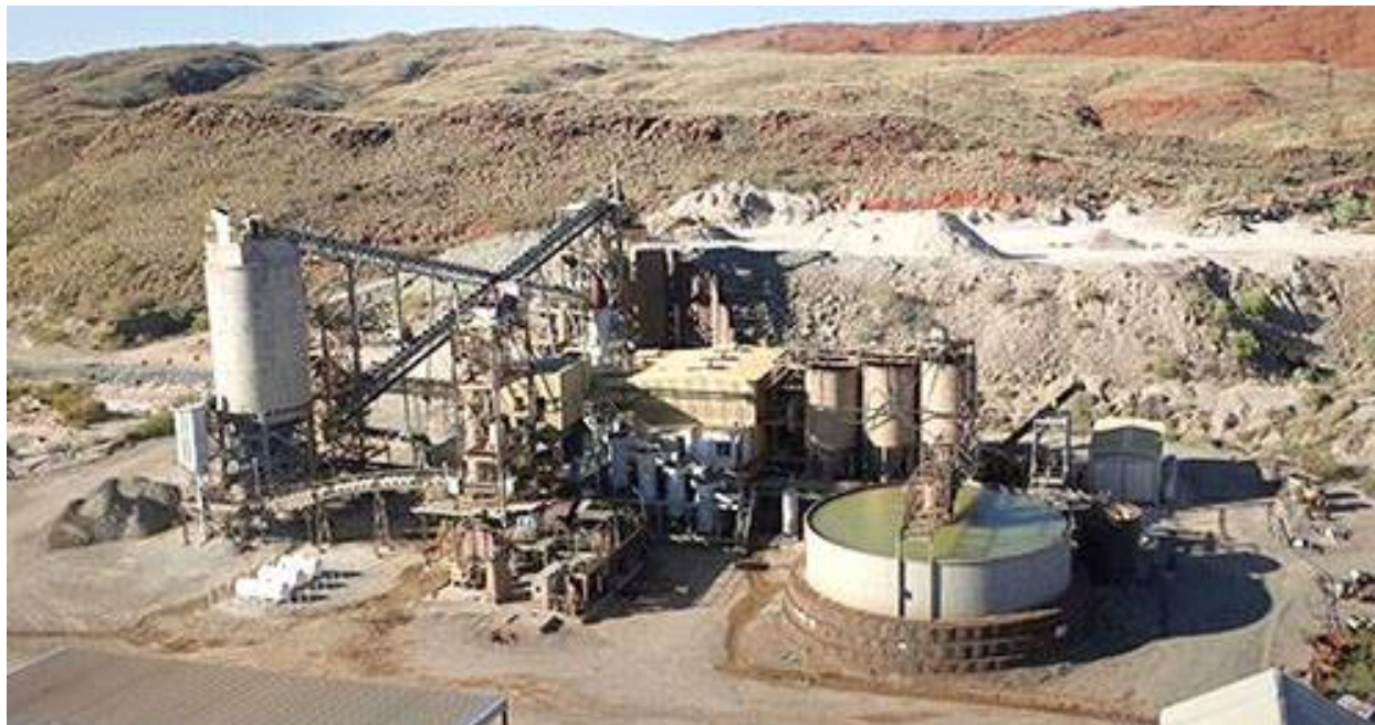
Figure 1: Bamboo Creek Processing Plant, Pilbara WA.
