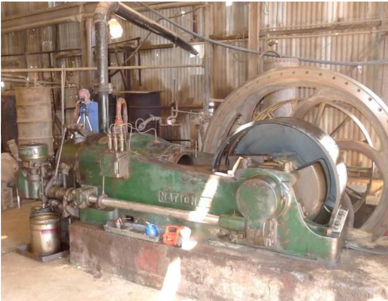
Figure 18: Comet Gold Mine National Diesel Power Engine.
