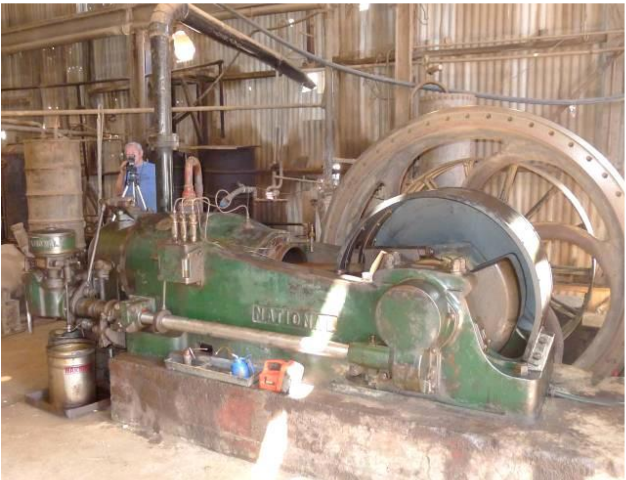
Figure 12: Comet Gold Mine National Diesel Power Engine
