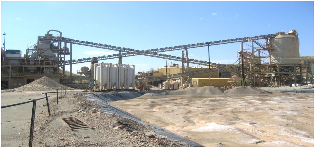
Figure 4: Bamboo Creek Processing Plant including Bamboo Creek Vat in the foreground containing 28,000 tonnes of crushed Kitchener Low Grade Ore sized '+180 microns to -3mm'
