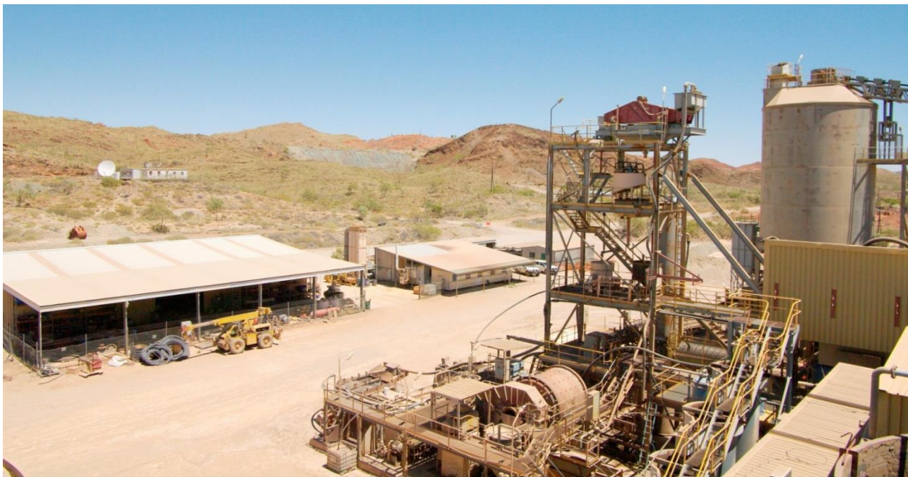
Figure 23: Bamboo Creek Processing Plant with the Tailings Dam Wall shown at top of the photo
