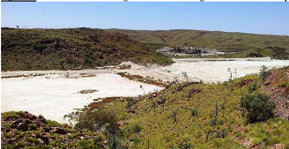
Figure 24: Bamboo Creek Tailings Storage with Bamboo Creek Processing Plant in background
