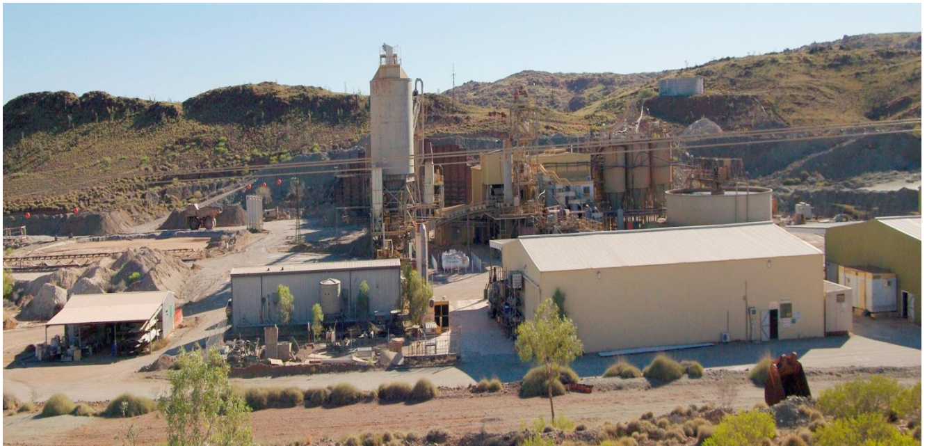
Figure 3: Bamboo Creek Processing Plant
