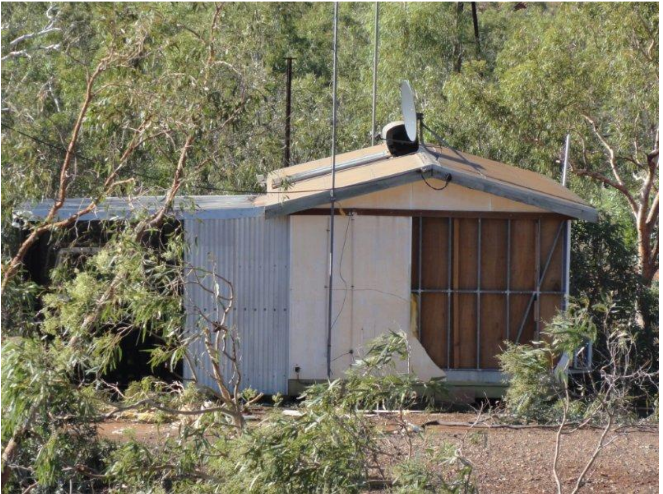
Figure 5: Tree and branch damage to accommodation
