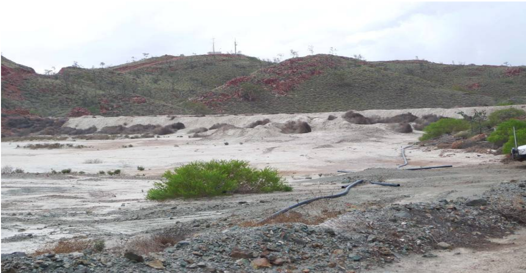
Figure 2: Bamboo Creek Tailings Dam
