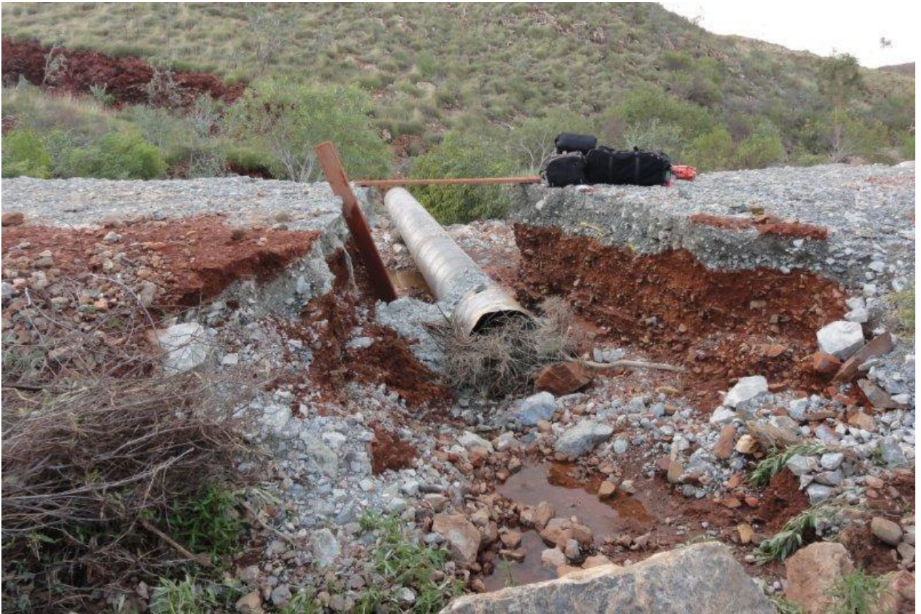
Figure 4: Bamboo Creek access road washed out
