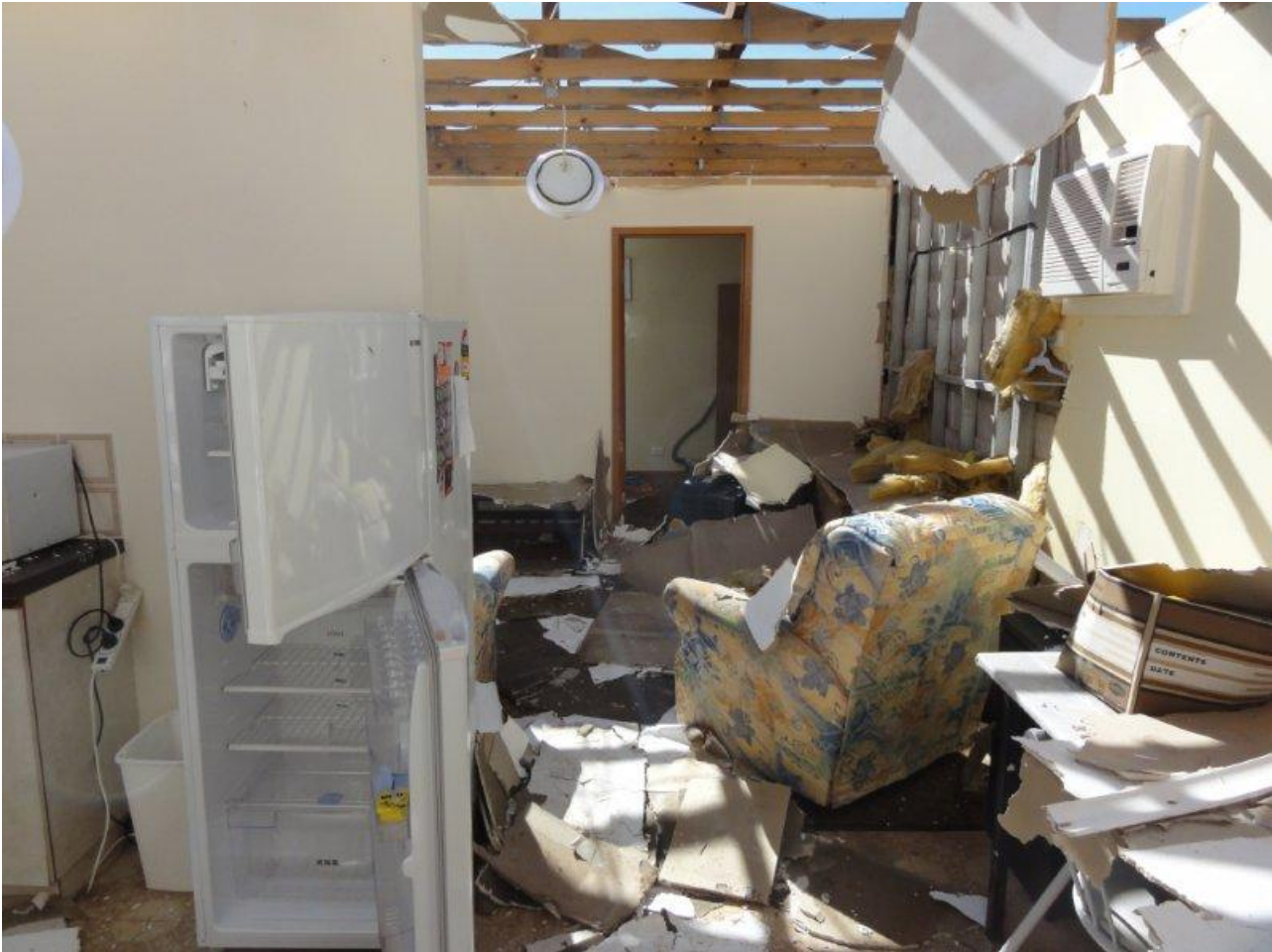
Figure 7: Internal damage to accommodation
