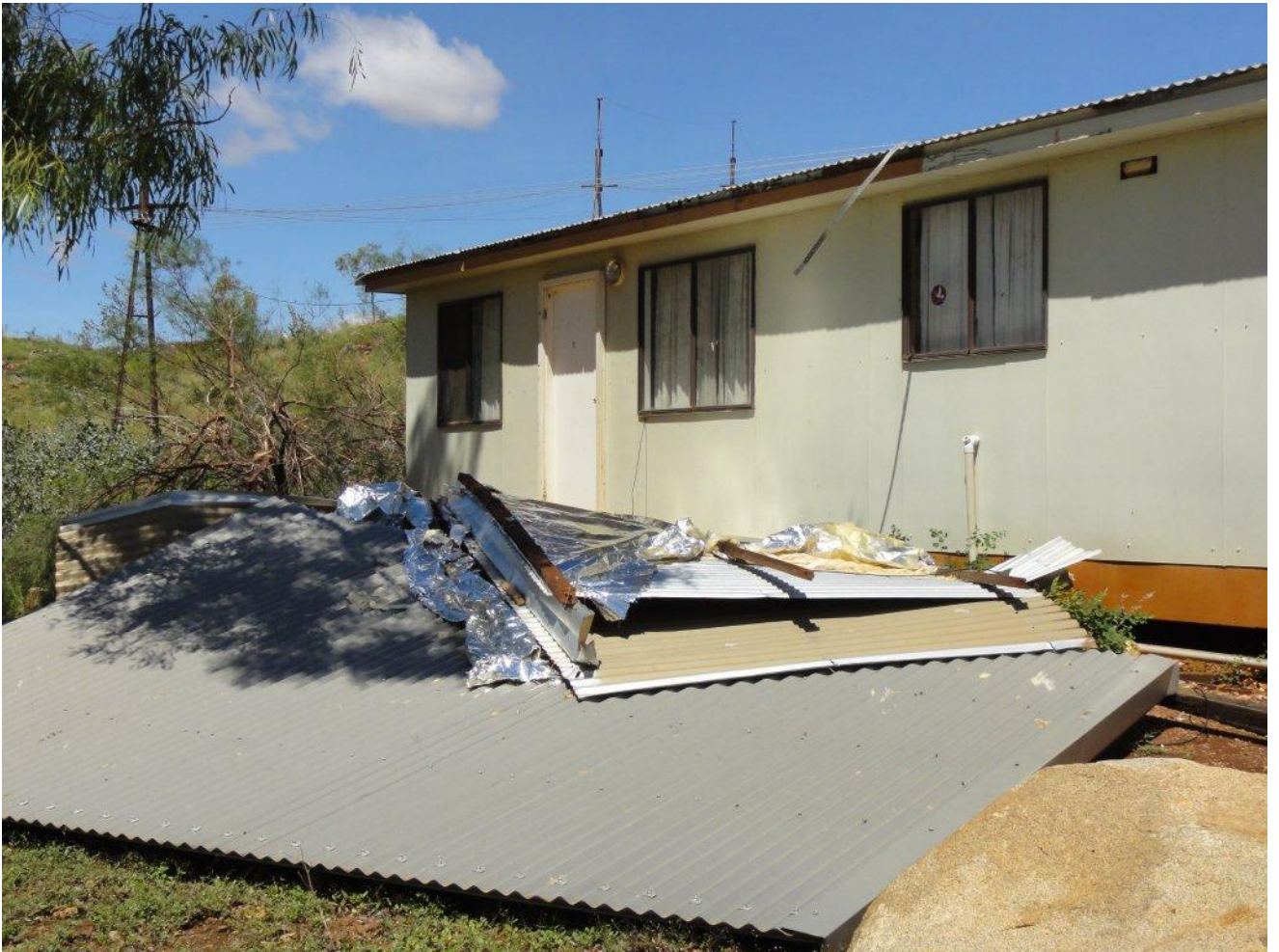
Figure 6: Dislodged roofing sheets
