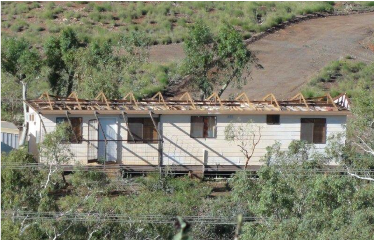
Figure 3: Unroofed staff accommodation
