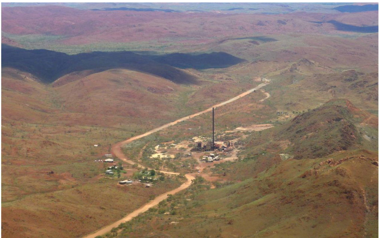
Figure 11: Comet Gold Tourist Centre and Comet Mine Plant (looking south) showing ore bearing ranges on right. Road goes to Mt Webber (approximately 80km)
