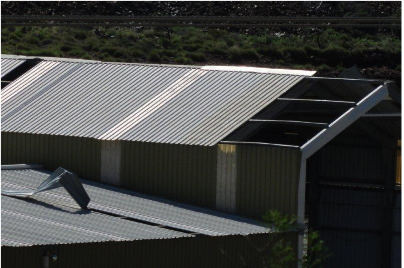
Figure 9: Roofing sheets blown off workshops
