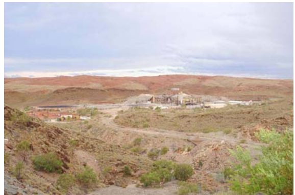
Bamboo Creek Plant from the Tailings Dam
