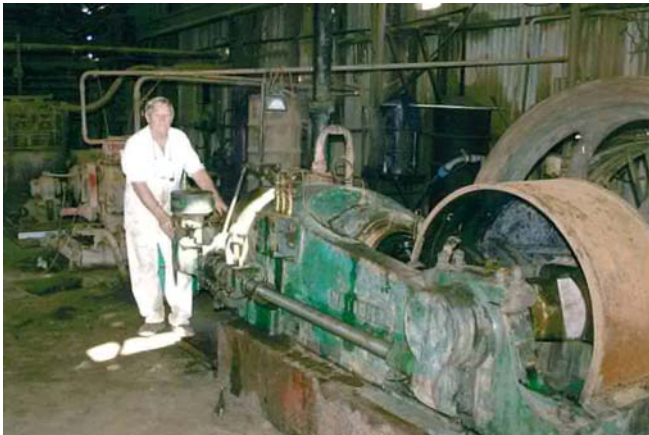
Comet Mine Power Station: Restored Single Cylinder NAW Diesel Engine, 66 horsepower & 300 rpm
