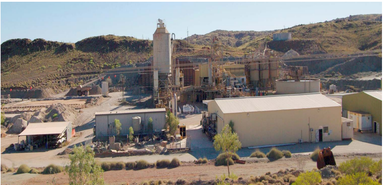
Figure 1: Bamboo Creek Processing Plant
