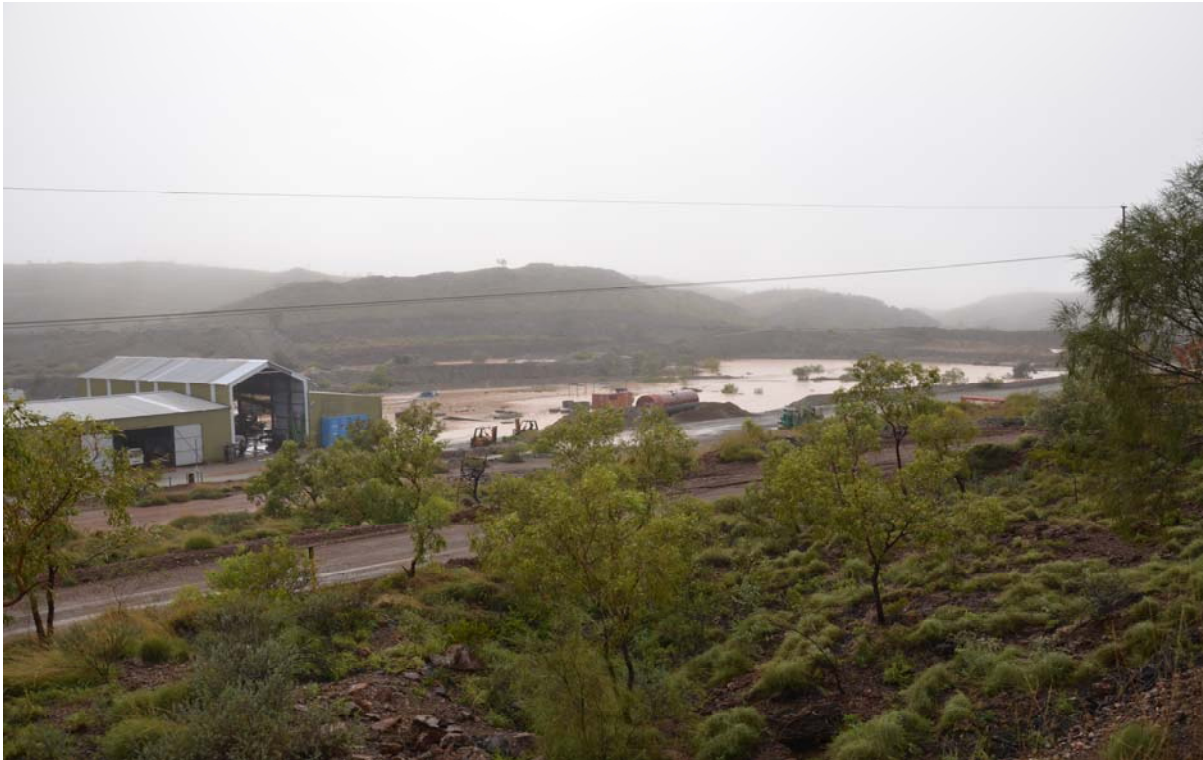
Figure 4: Flooding at Bamboo Creek Pilot Plant from Tropical Cyclone Rusty
