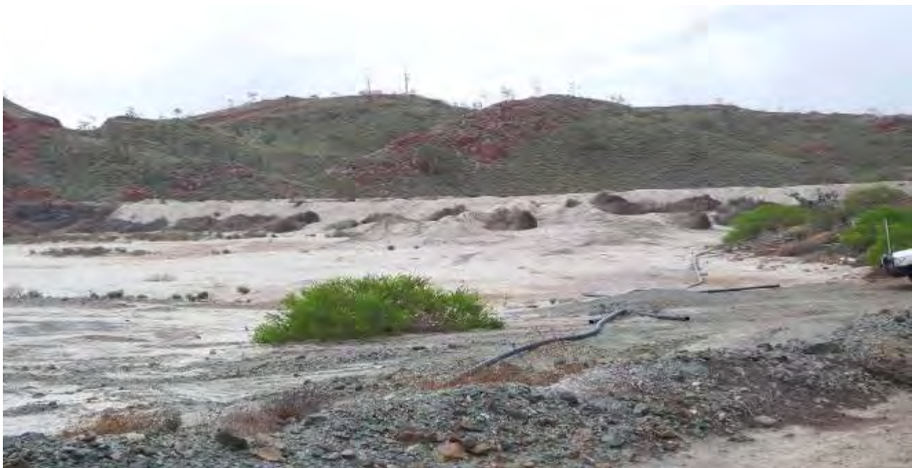
Figure 3: Bamboo Creek Tailings Dam
