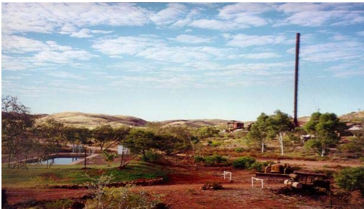
Comet Gold Mine Plant from Tourist Centre
