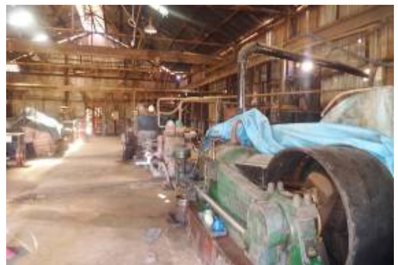
Figure 16(s): Comet Mine Power Station
