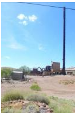
Figure 16(b): Comet Mine 'Stack' & Plant
