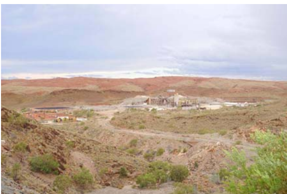
Figure 3(h): Bamboo Creek Plant from
