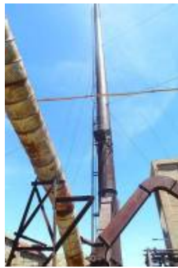
Figure 16(c): Comet Mine 'Stack'
