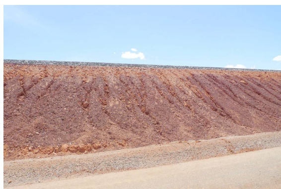
FMG Railway Line Embankment
