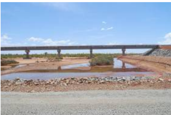
FMG Railway Line at Turner River Crossing
