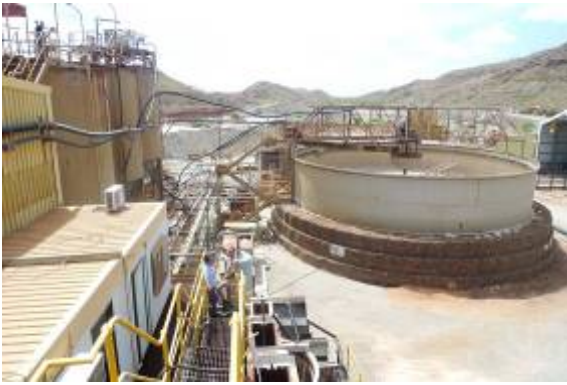
Bamboo Creek Plant Leach Tanks and Thickener
