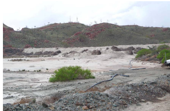
Bamboo Creek Tailings Dam
