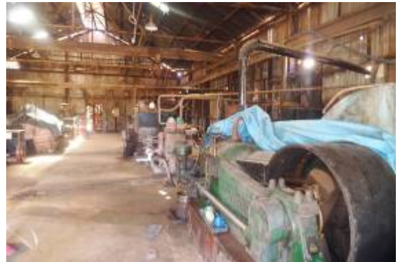
Comet Mine Power Station
