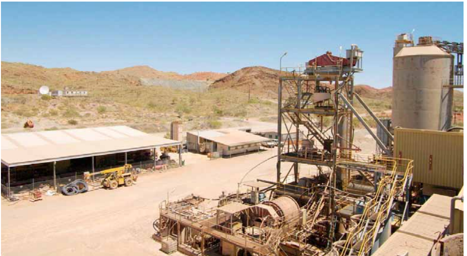
Bamboo Creek Processing Plant with the Tailings Dam Wall shown at the top of the bottom photo.
