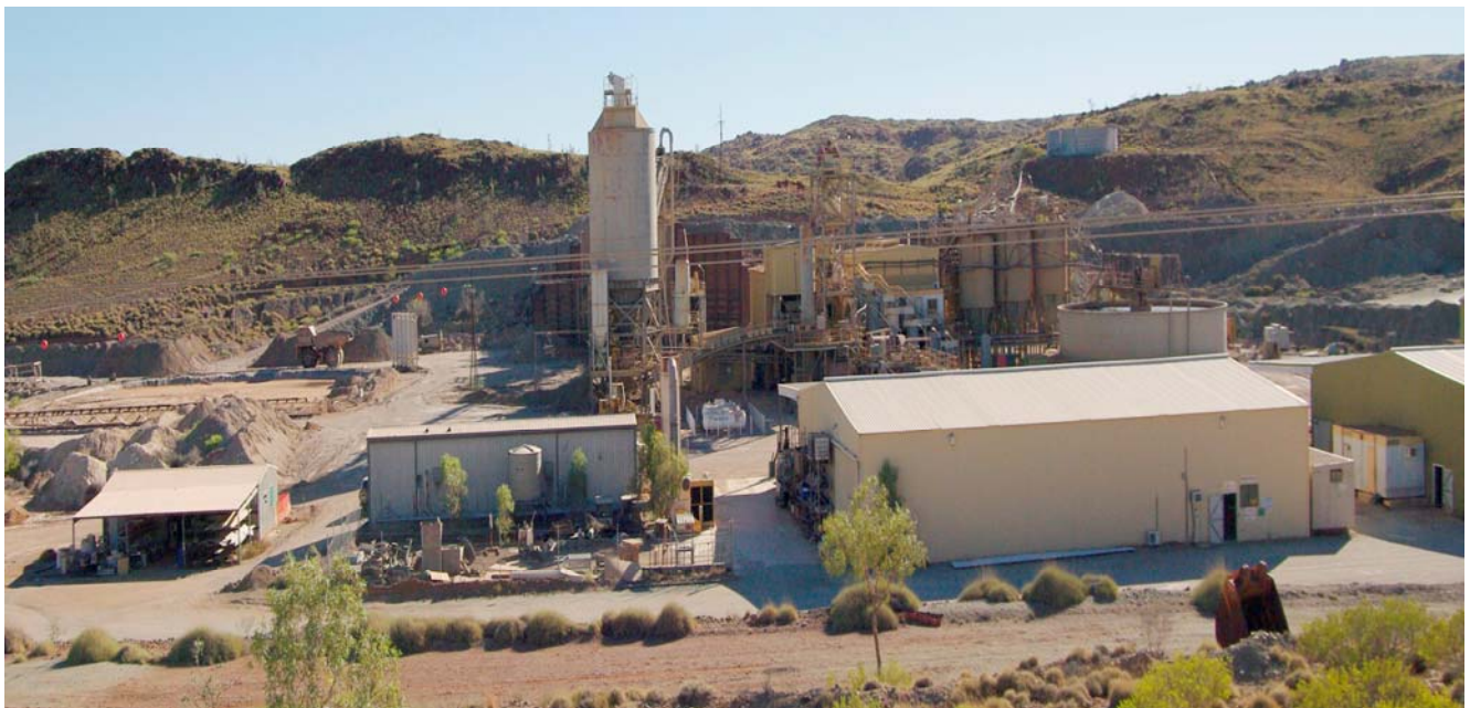
Figure 1: Bamboo Creek Processing Plant
