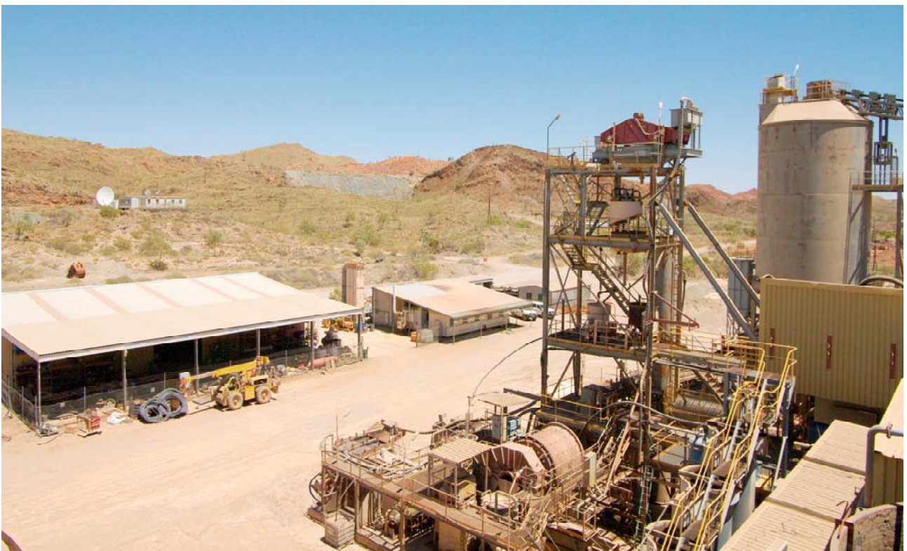
Figure 5: Bamboo Creek Processing Plant with the Tailings Dam Wall shown at the top of the photo
