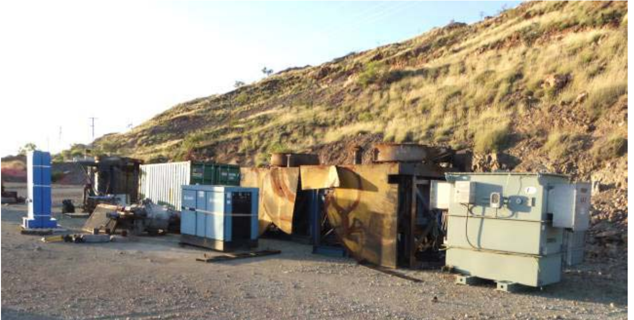
Figures 16 & 17: Three 3 tonne Induction Furnaces recently purchased and soon to be installed in the upgraded Bamboo Creek Plant
