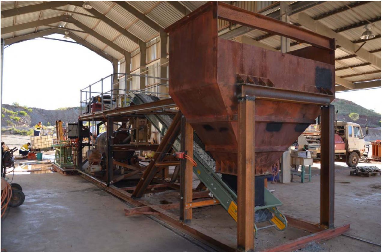
Figure 8: Hopper ore ‘bin’ used to feed Conveyor to Ball Mill
