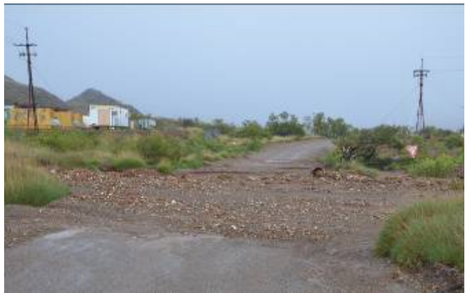
Figures 3 & 4: Bamboo Creek roads ‘washed out’ following Tropical Cyclone Rusty
