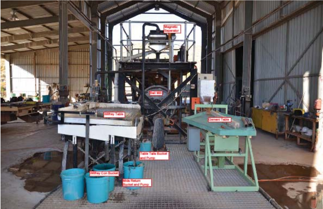
Figure 7: Bamboo Creek Pilot Plant
