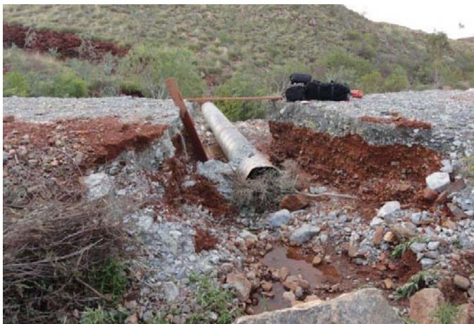
Figure 6: Bamboo Creek access road washed out
