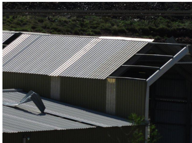
Figure 7: Roofing sheets blown off workshops
