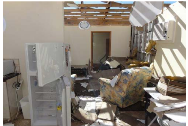
Figure 5: Internal damage to accommodation
