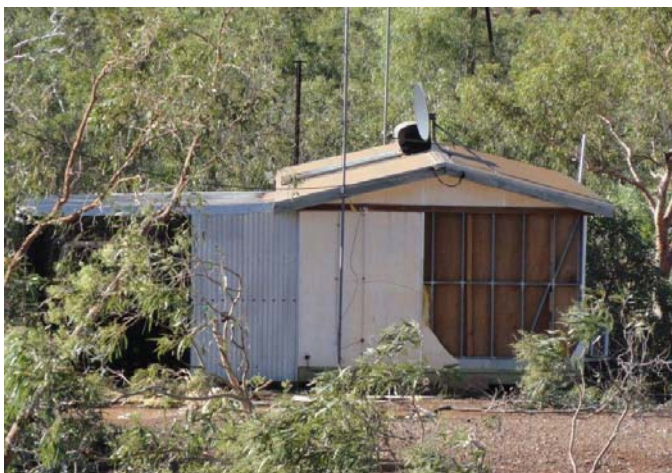
Figure 8: Tree and branch damage to accommodation
