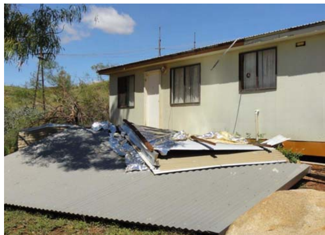
Figure 9: Dislodged roofing sheets
