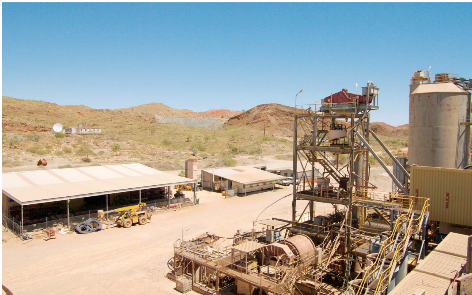
Bamboo Creek Processing Plant with the Tailings Dam Wall shown at the top of the bottom photo
