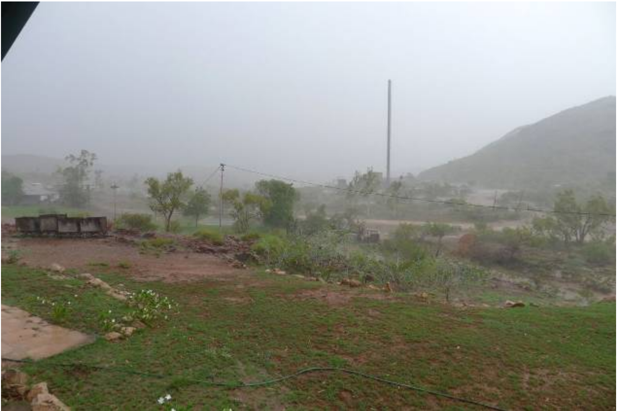
Figure 12: Comet Gold Mine Plant from Tourist Centre during heavy rain caused by cyclone activity in the Marble Bar area
