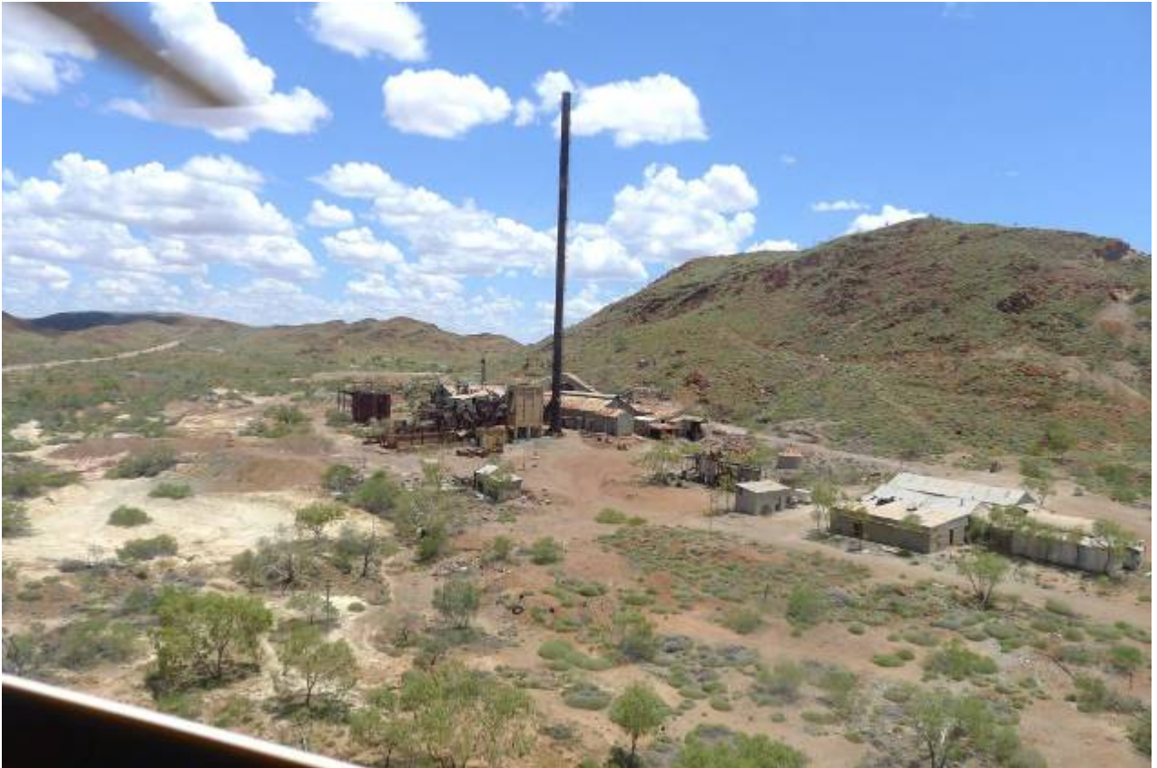
Figure 11: Close-up of Comet Gold Mine Plant with ore bearing range behind
