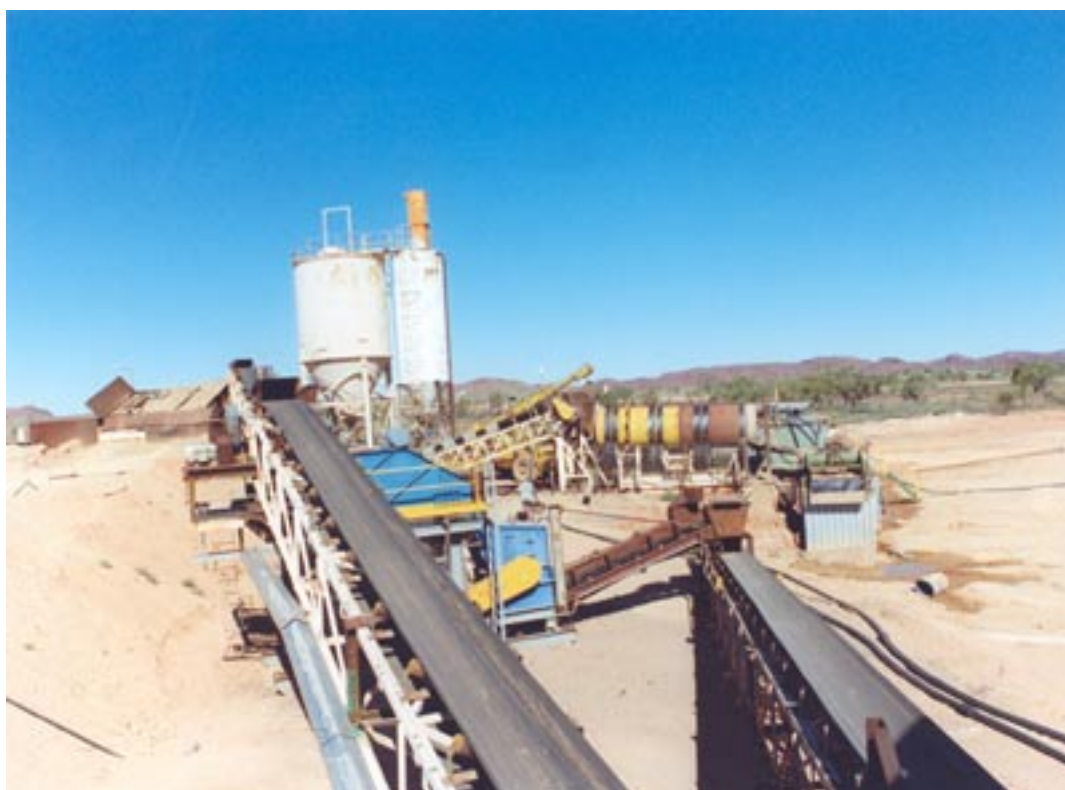
Normay Processing Plant Pilbara, WA
