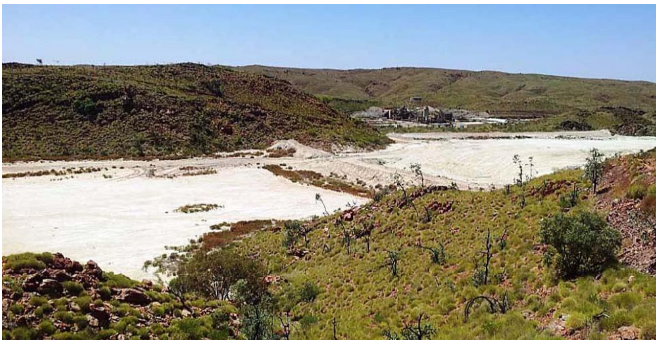
Figure 18: Bamboo Creek Tailings Storage with Bamboo Creek Processing Plant in background
