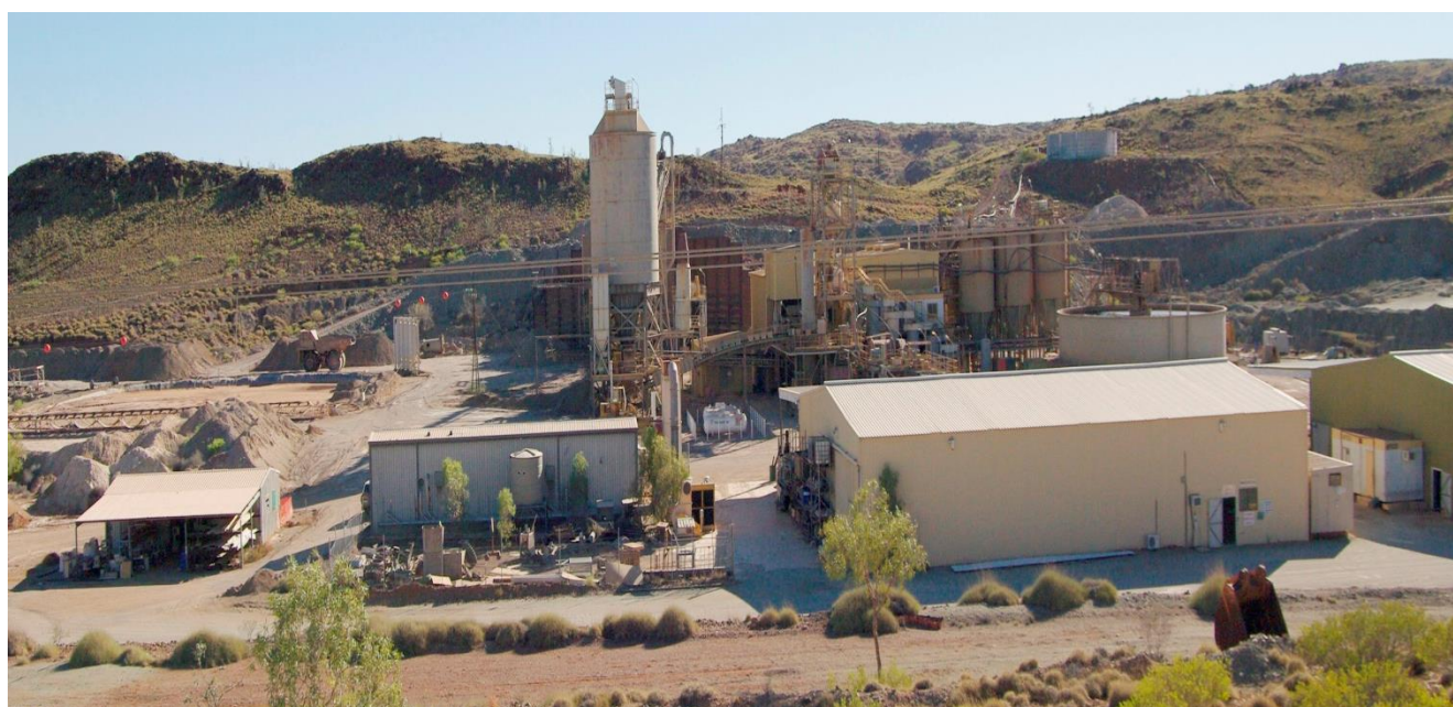
Figure 20: Bamboo Creek Processing Plant looking north, Conglomerate Formations behind range.
